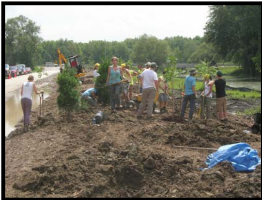
Planting on river relocation project in Holland Marsh
