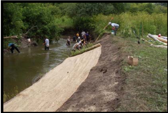
Erosion control project on Little Rouge Creek
