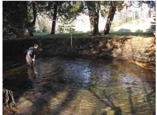
Photo 2: Steep eroding bank opposite man-made rock weir
