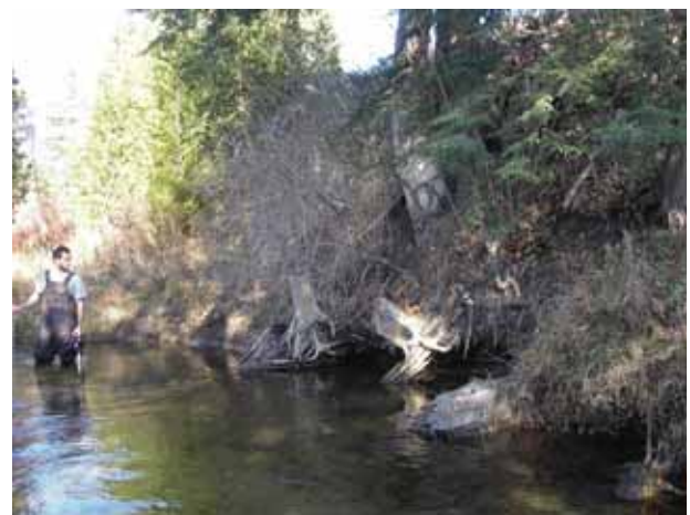
Photo 6: Steep eroding bank; debris jam recommended
