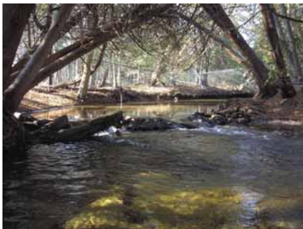
Photo 3: Man-made rock weir causing downstream erosion
