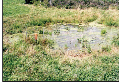
This simple “Hickenbottom” can be a cost-effective method for restoring small wetland areas.
